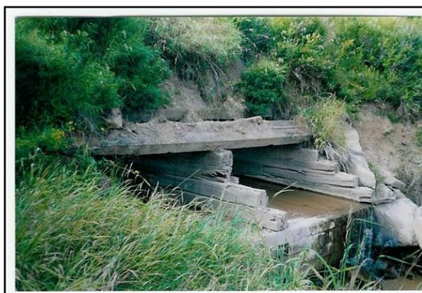
**Figure 2:** Close up of the old, double chambered, wooden culvert (CCCB 13C) at Christie Brook (River Hebert, NS). Classification: partial restriction. (Hynes et al., 2005)
