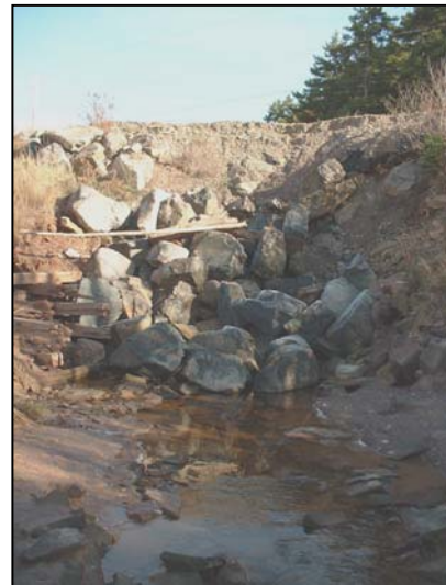
Figure 9. Upstream side of the culvert is damaged and collecting debris.
