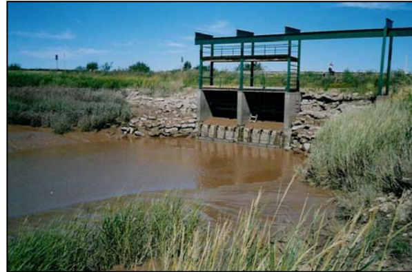
Figure 13. Downstream view of crossing
