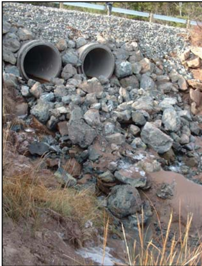
Figure 2. Double hanging culverts along the River Hebert
