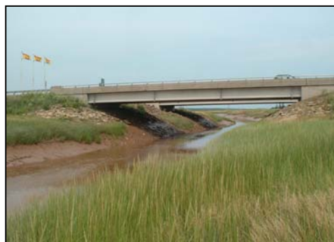
Figure 3. Highway bridge across the Missaguash River.
