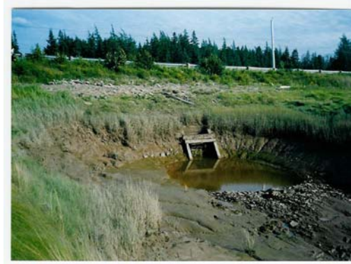
Figure 4. Mill Creek causeway-aboiteau (CCCB18A)
