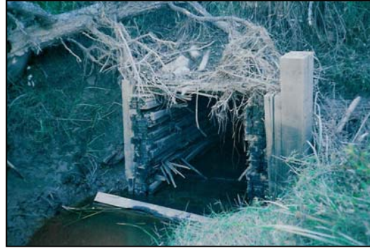
Figure 9. Upstream side of the culvert is damaged and collecting debris.
