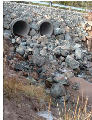
Figure 15. Downstream view of the new culverts.
