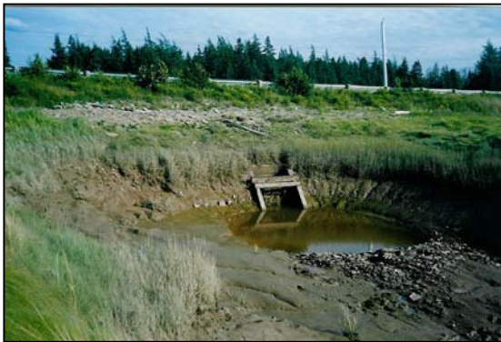
Figure 11. The downstream view of the causeway-aboiteau showing the scour pool and bank erosion.
