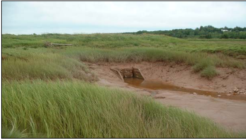
Left: main tidal channel, dyke and double aboiteau at low tide.
