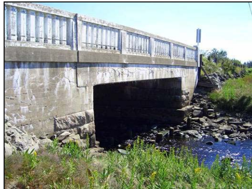
Figure 31. Downstream end of DC31B, slightly pinching river channel.
