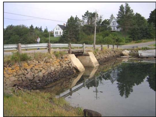
Figure 29. Downstream end of crossing, much smaller than the width of the river.
