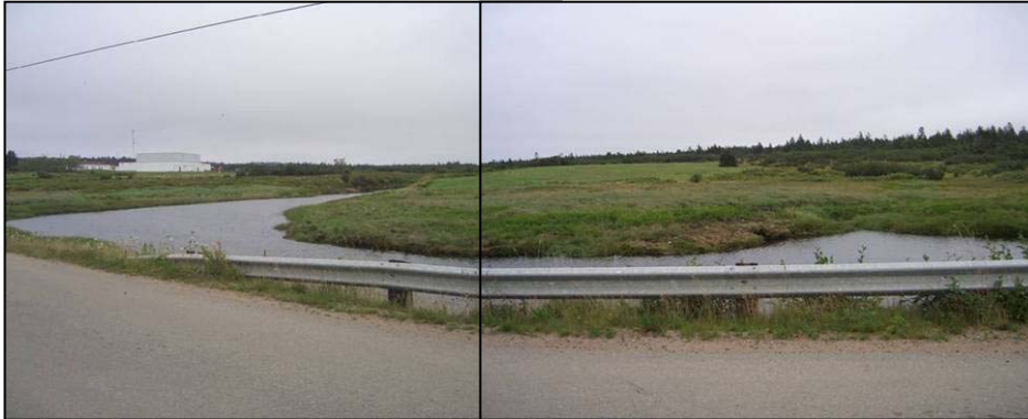
Figure 28. Upstream system looking from on top of the culverts.
