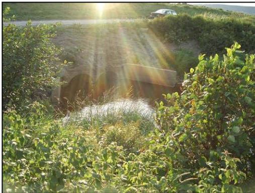
Figure 15. Upstream end of aboiteaux
