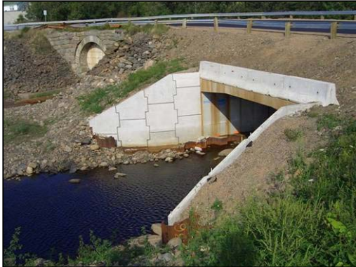
Figure 9. Downstream end of the new culvert.
