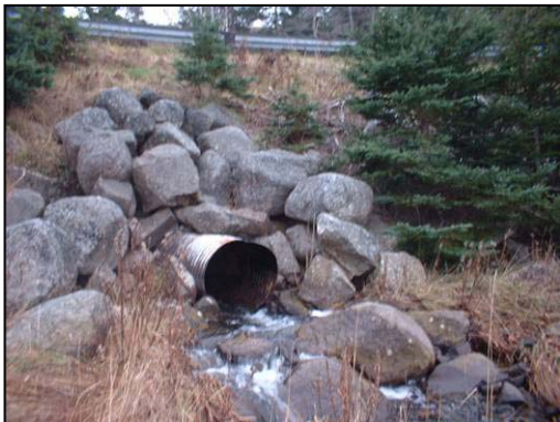
Figure 10. Downstream end of rail bed; culverts completely collapsed (DC6C).
