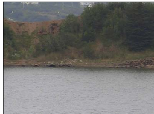
Figure 24. Rail bed crossing, looking from the upstream crossings.
