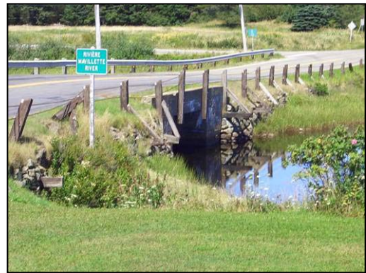
Figure 20. DC43B – Mavillette River, upstream end.
