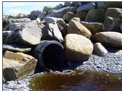
Figure 35. Downstream end of aboiteau covered by large boulders.
