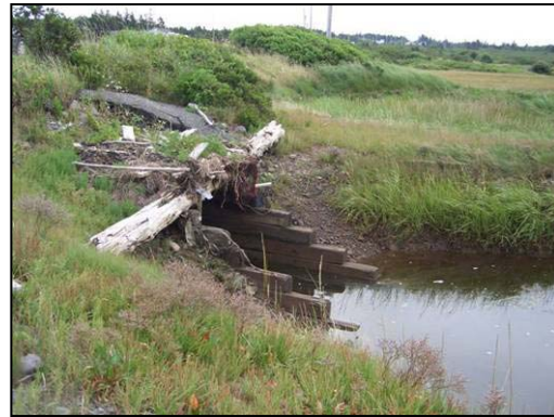
Figure 14. Downstream end of culvert
