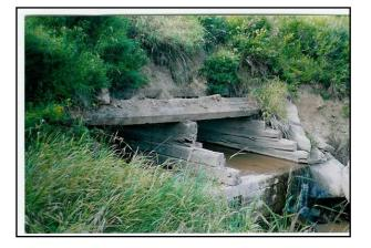
*Figure 2:* Close up of the old, double chambered, wooden culvert (CCCB 13C) at Christie Brook (River Hebert, NS). Classification: partial restriction.(Hynes et al., 2005)
